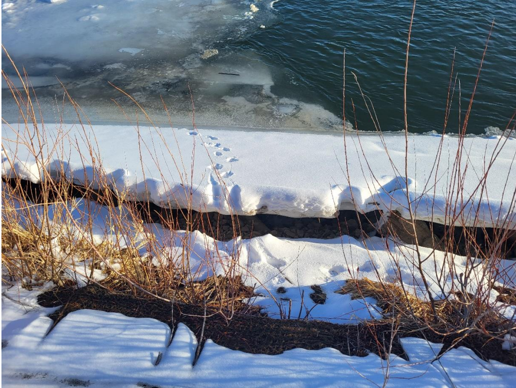
Ice slab pushing over wood toe, no damage viewed at this time
