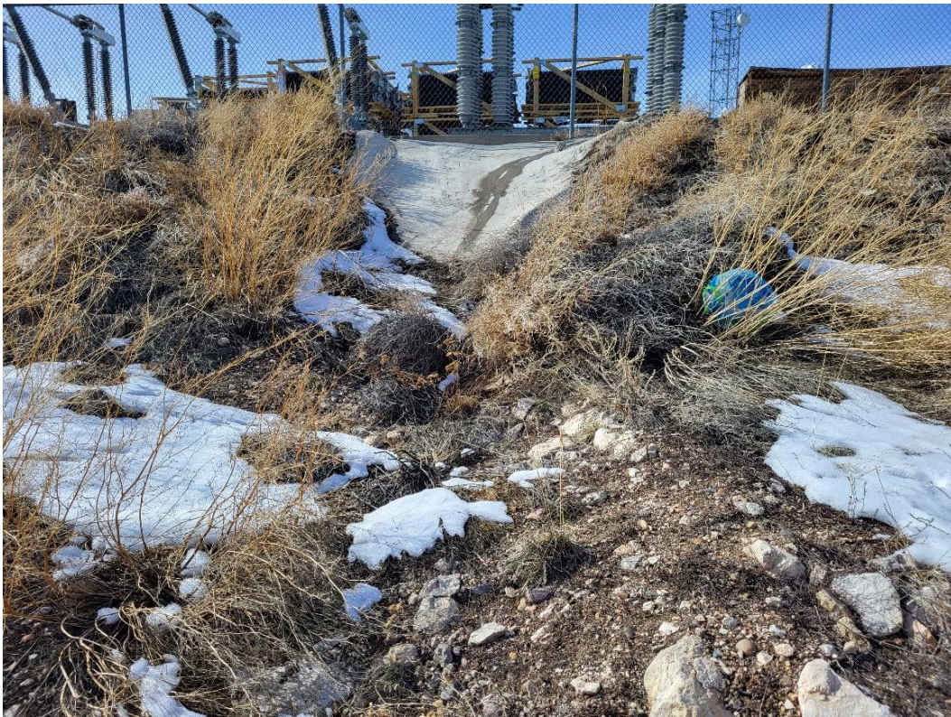
Concrete apron below utility yard river left sta. 22+50
