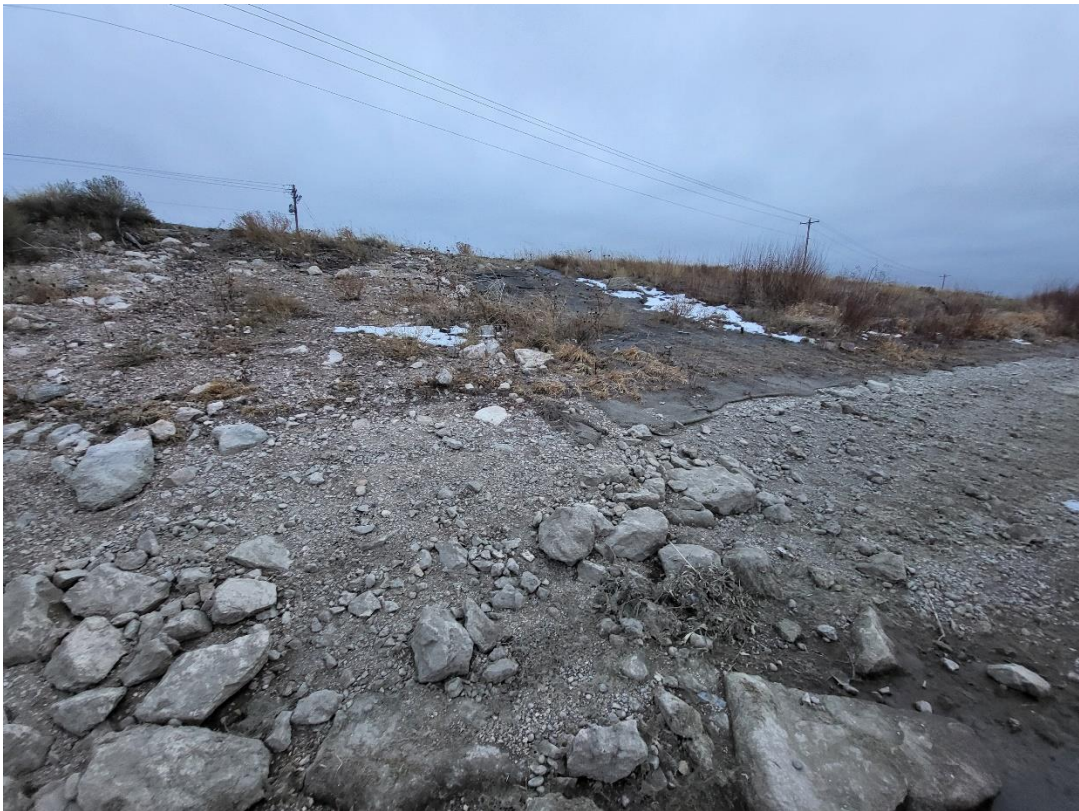
Access ramp, below staging area
