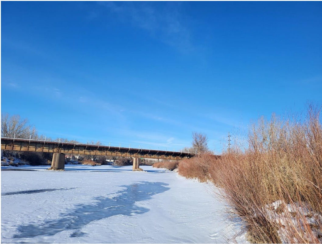
Looking downstream at BNSF bridge
