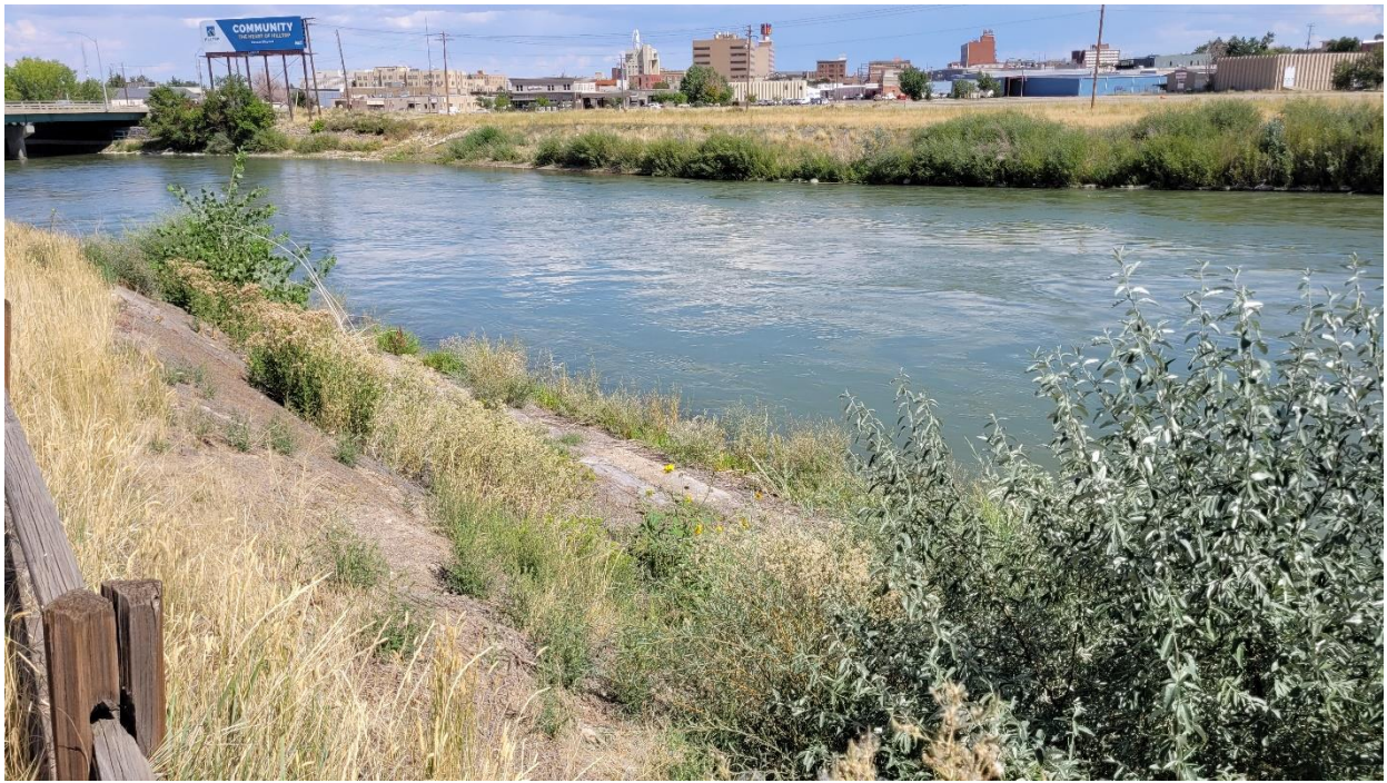
Willow stakes in first burrito rap growing, willows in second burrito rap did not survive. View looking generally downstream, 1 st Street Bridge in upper left of photo.
