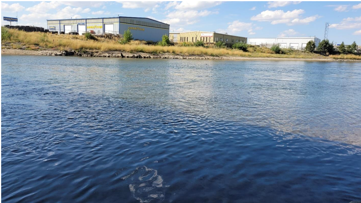
View of river left, in the vicinity of the Goodyear building, showing apparent erosion area noted in previous photo. Eroded area is just right of smooth stream bank visible in far left of photo. Monitoring wells just visible in grass above the area. Note that this area had eroded significantly prior to construction – the bank was eroded back to the monitoring wells. Also note general absence of vegetation along bank to right of photo.
