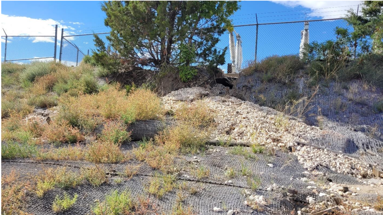
River left, downslope from power company yard. Note white gravel placed since construction, on top of burlap, to fill in bank erosion, apparently from runoff from paved area above.
