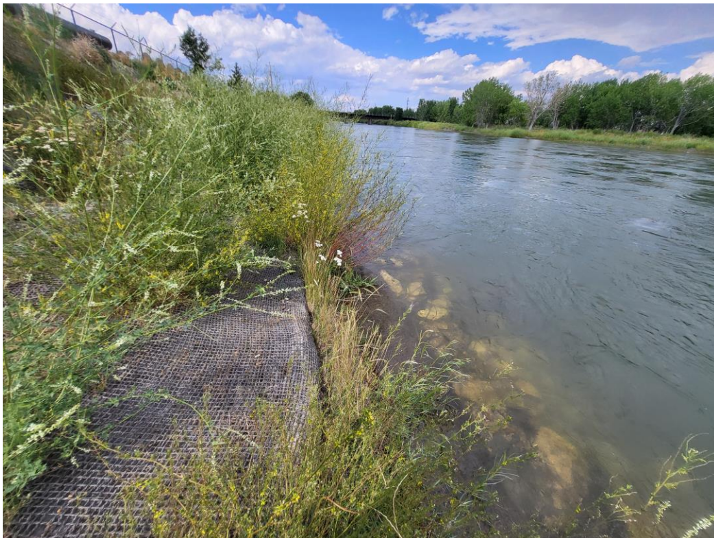
River left from sta 17+00 to BNSF Railroad, 70% coverage with a majority of weeds
