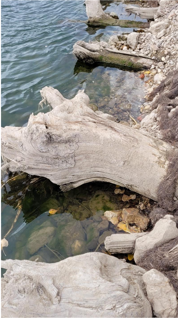
View of woody toe looking upstream, river left, just upstream of Jonah Bank building. Note gravel bed up to bottom of woody toe, no apparent undercutting of woody toe.
