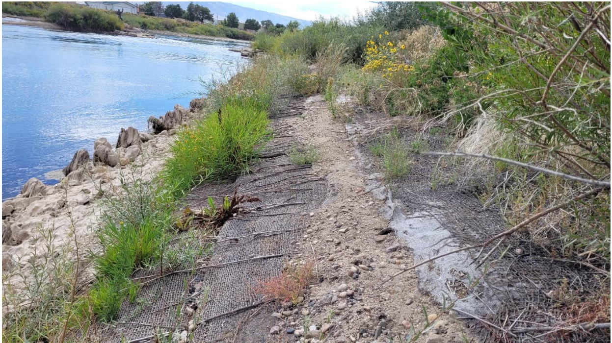
View of river left bank just below fisherman statute, visible in upper left of photo. Note some grasses and willows establishing along high water level, general absence of vegetation just above that level.
