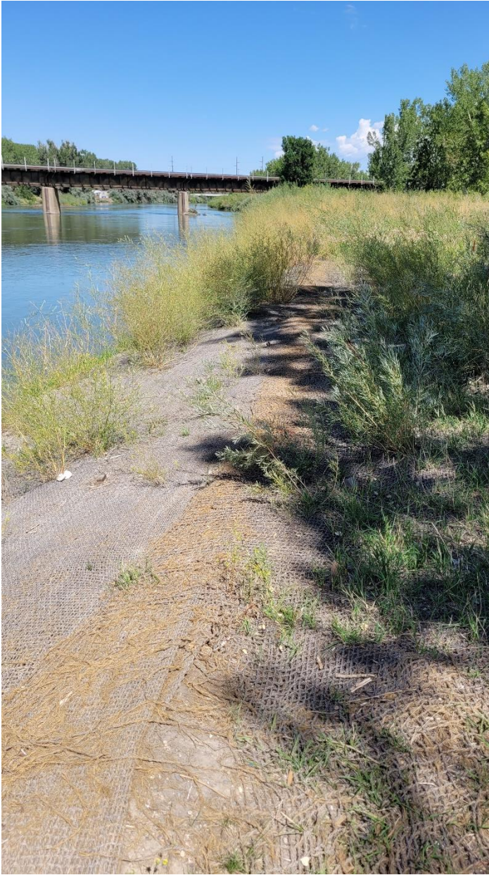
Limited vegetation river right, approximately Sta. 23+00.
