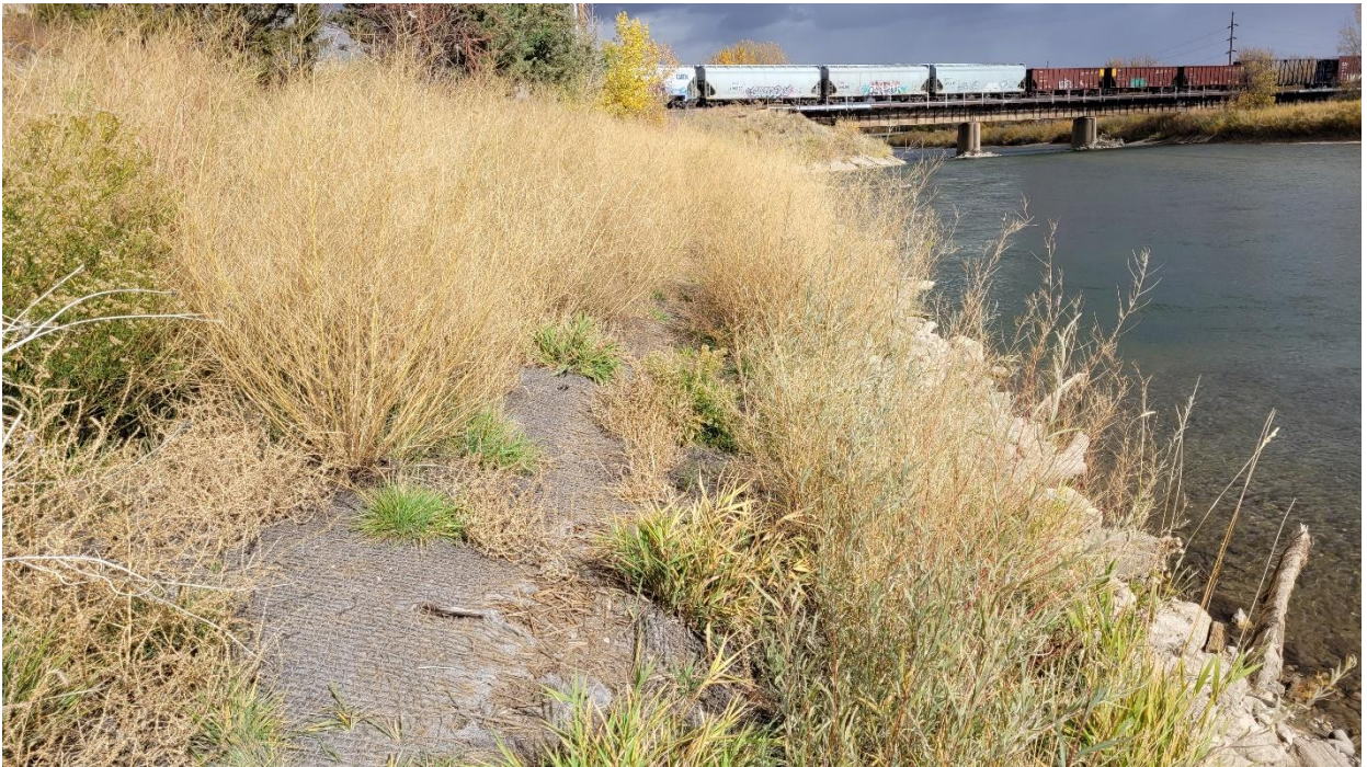
View looking downstream from river left, note BNSF railroad bridge in upper right of photo. Note grasses and willows along water line to right, with barren areas in next burrito wrap away from riverbank. Much of vegetation present is weedy in nature.
