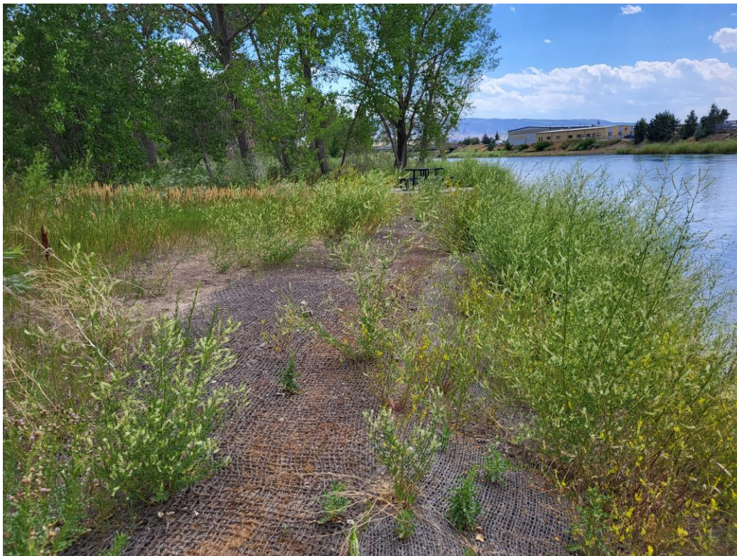
Limited vegetation river right, approximately Sta. 23+00
