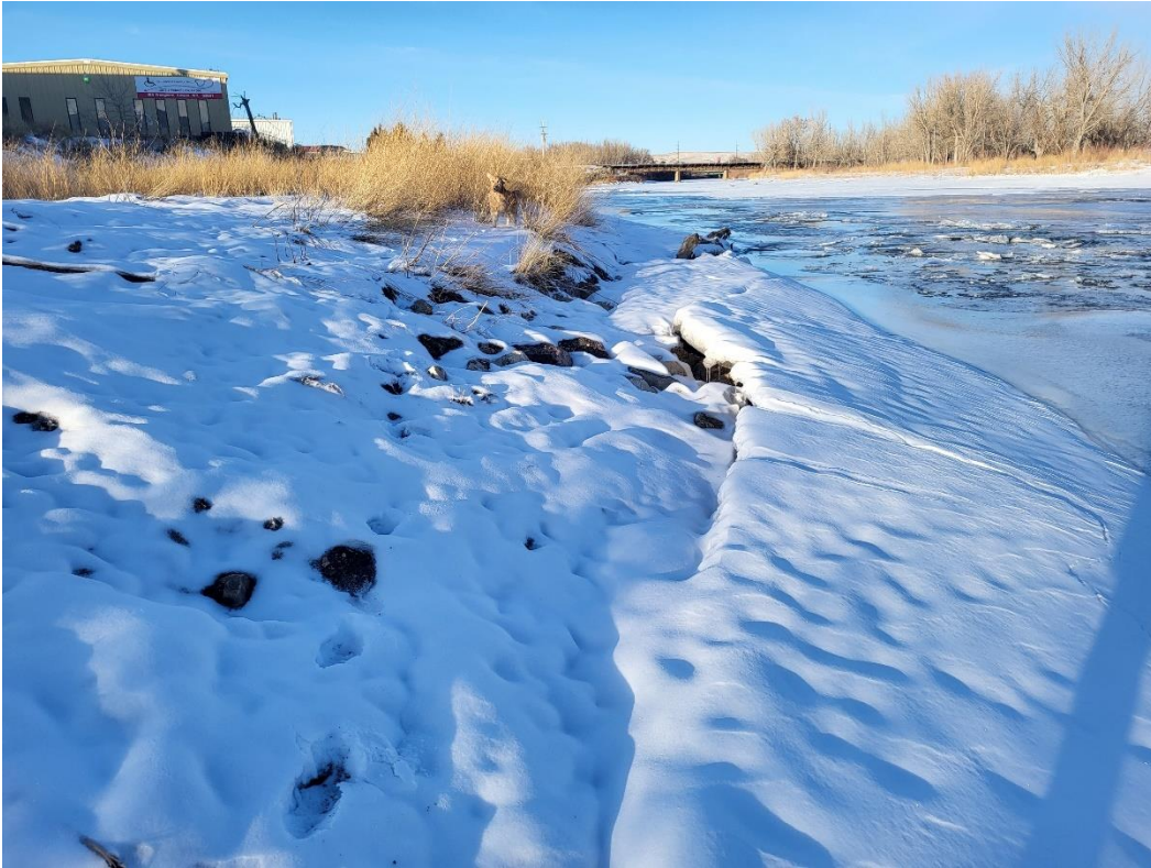
River left, just downstream of First Street Bridge, adjacent to the three monitoring wells
