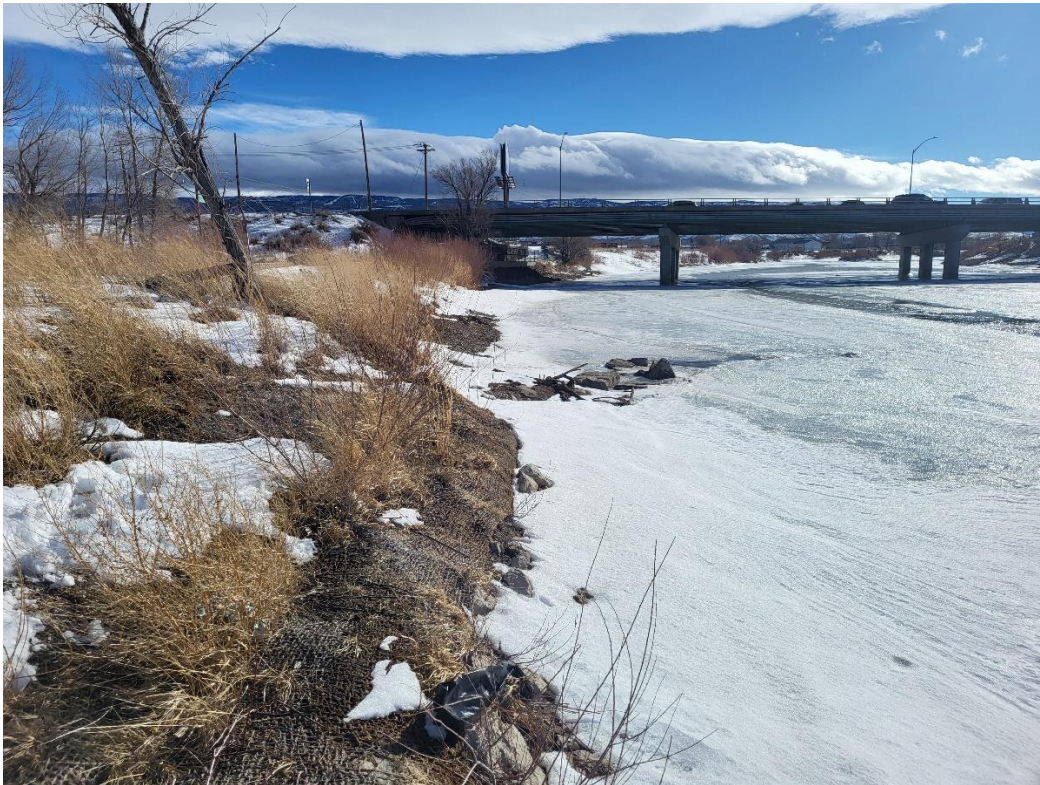
J-Hook structure starting to become visible through the snow and ice river right sta. 16+00
