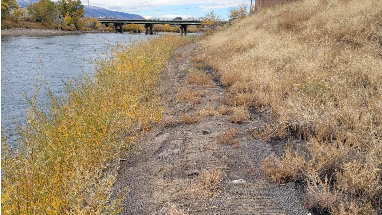
River left, looking upstream, from Jonah Bank area, 1 st Street bridge in upper center of photo. Willow stakes in first burrito established, second burrito rap willow stakes did not grow. Note generally sparse vegetation in second burrito wrap.
