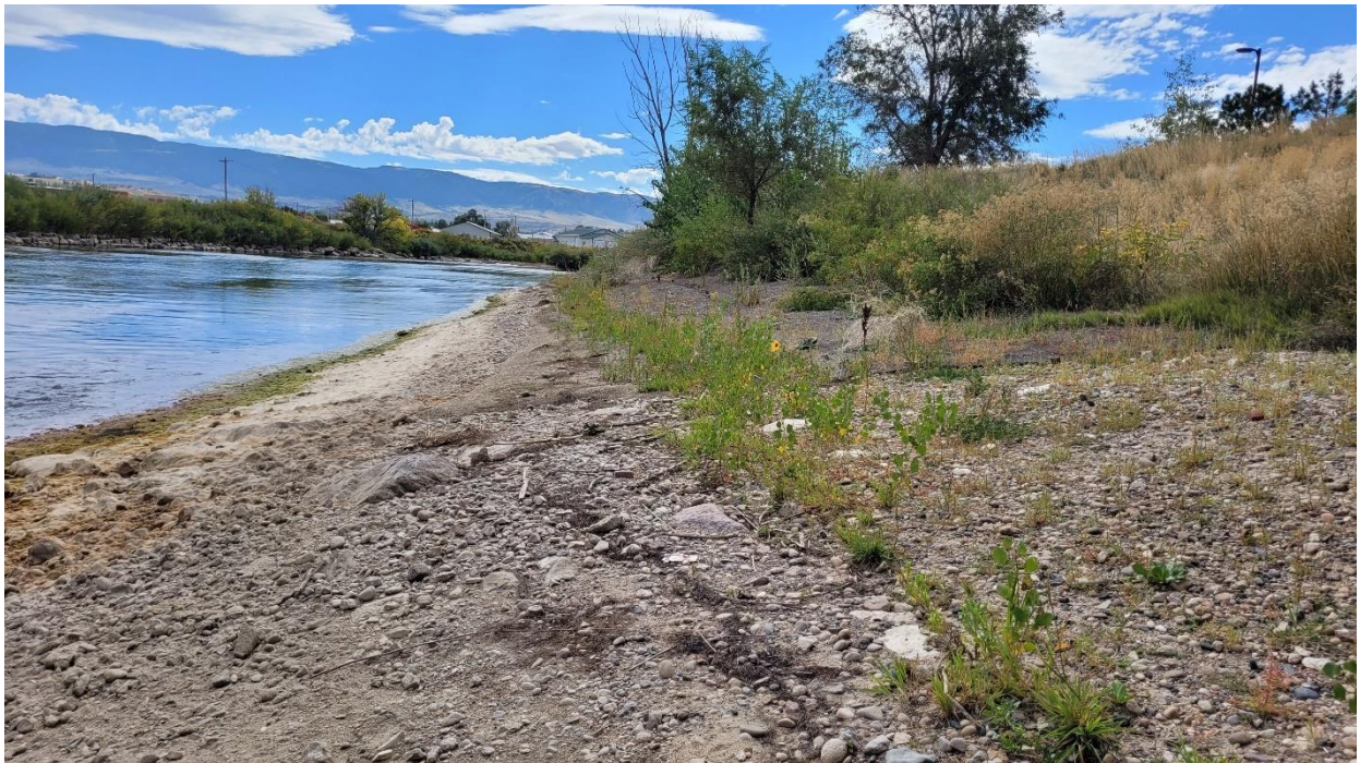
View river left, looking upstream from 1 st Street bridge. Note line of vegetation establishing along high water line, but sparse vegetation otherwise in construction area.
