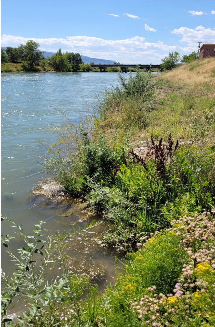
River Left, looking upstream, 1 st Street bridge in upper center of photo. Willow stakes in first burrito established, second burrito rap willow stakes did not grow.
