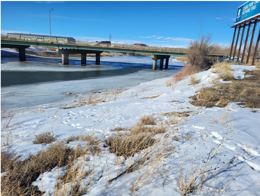
Access ramp, river right sta. 12+00
