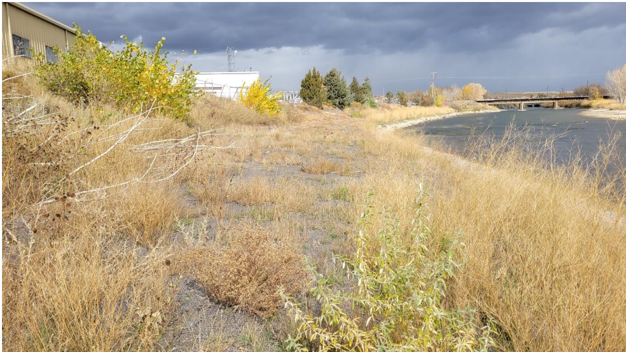
River left, looking downstream, All About Family Inc. building visible in upper left of photo. Note weedy nature of vegetation, and Russian olive regrowth in foreground. Vegetation is predominantly weeds, actual coverage by grasses and willows, etc. is limited.
