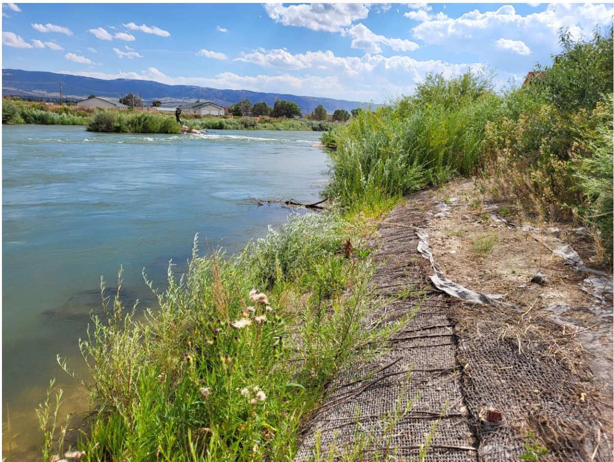
Willow stakes in first burrito rap growing, willows in second burrito rap did not survive
