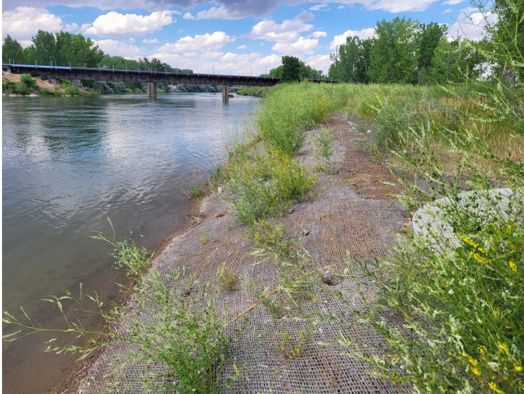
Limited vegetation river right, approximately Sta. 23+00
