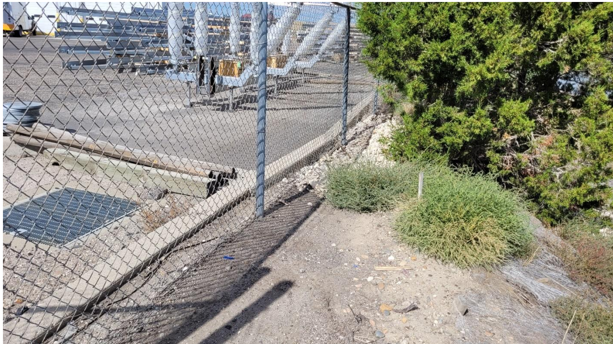
View of edge of electric company yard, in area where runoff apparently overflows curb during some storm events. Note similar white gravel as in previous photo along fence.
