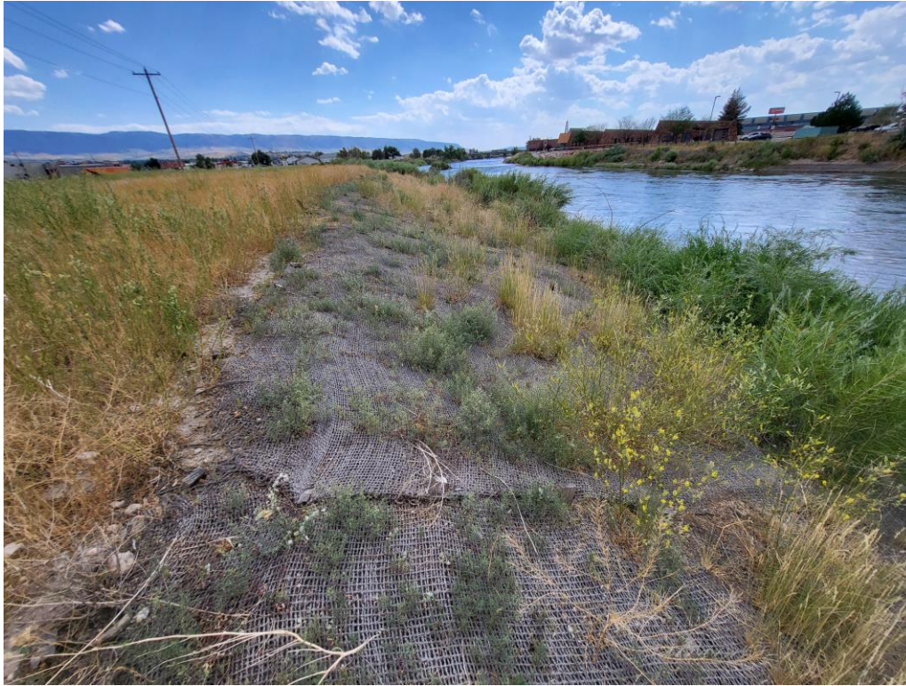
River bank slope adjacent/south of access ramp river right, willows next to rivers edge established. Away from rivers edge is 10 to 20% coverage.
