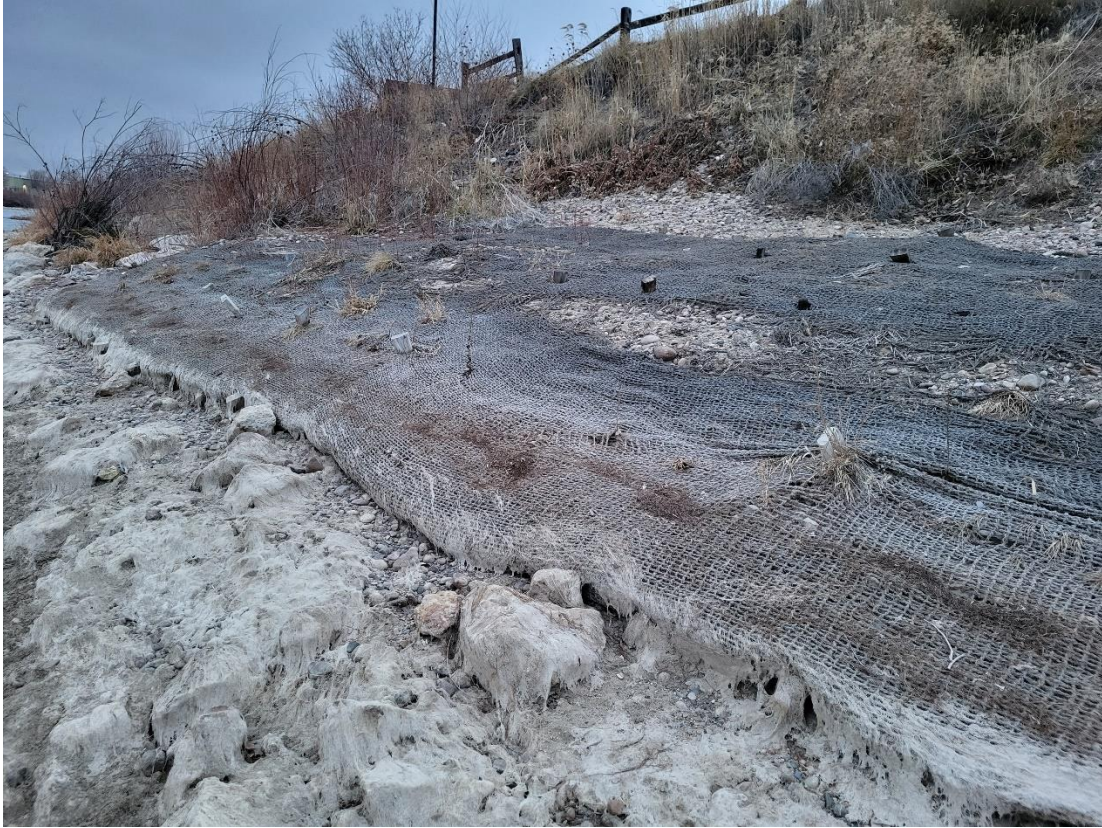
Sparse vegetation river, left just upstream from 1 st Street Bridge
