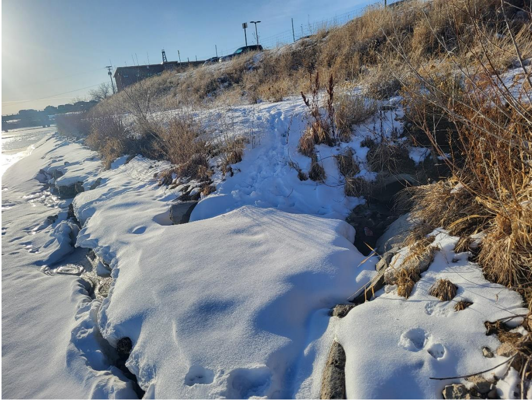
Ice jam and outlet structure
