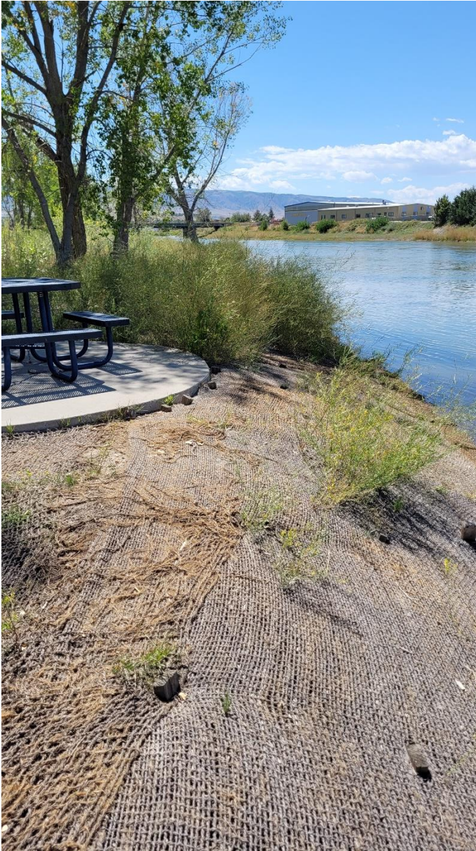
Limited vegetation river right, approximately Sta. 23+00.
