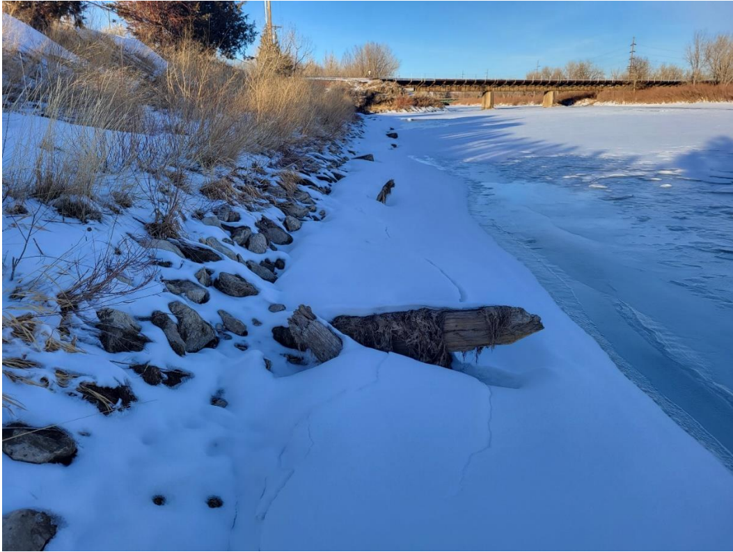
River left, looking downstream at BNSF Bridge
