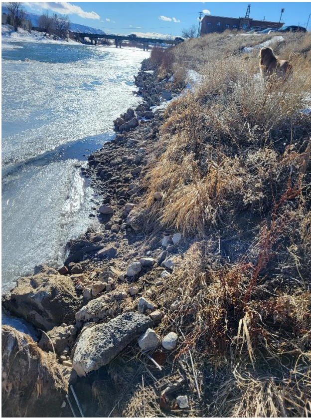
Small erosion area river left sta. 4+75, just upstream of outlet structure
