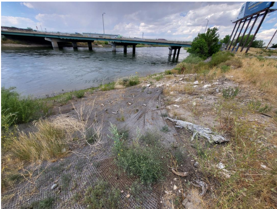
Vegetation on construction access ramp is approximately at 10% coverage
