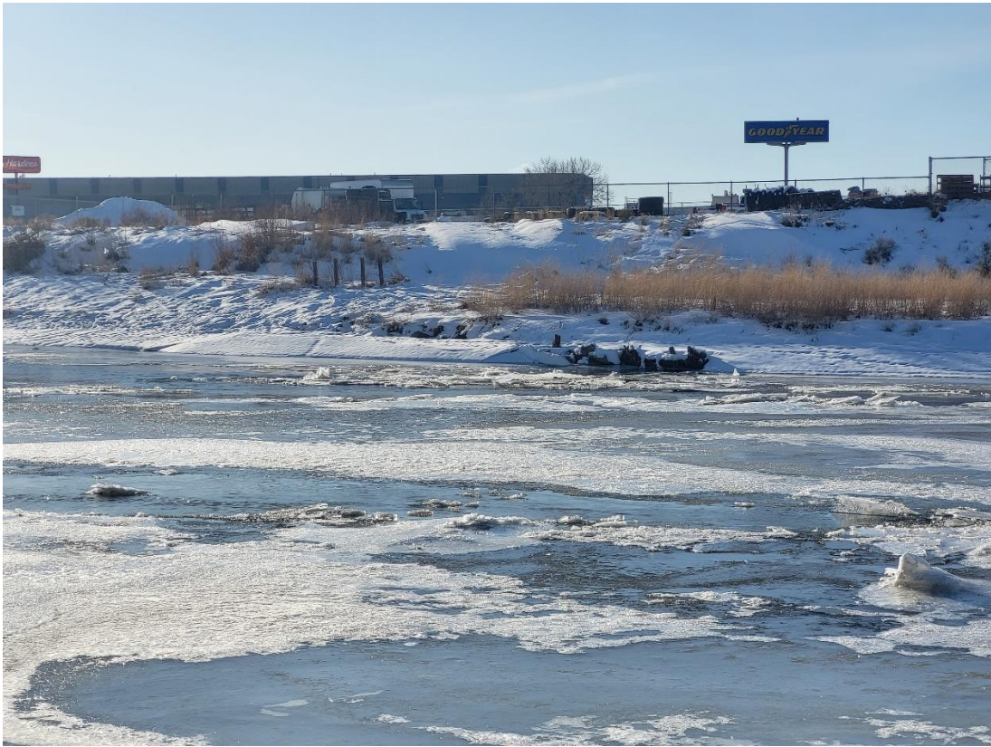
Repaired erosion area, river left
